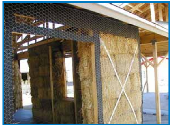
Straw bale construction provides an innovative way to build affordable green homes and preserve the environment. Photo provided by Tierra Madre.
